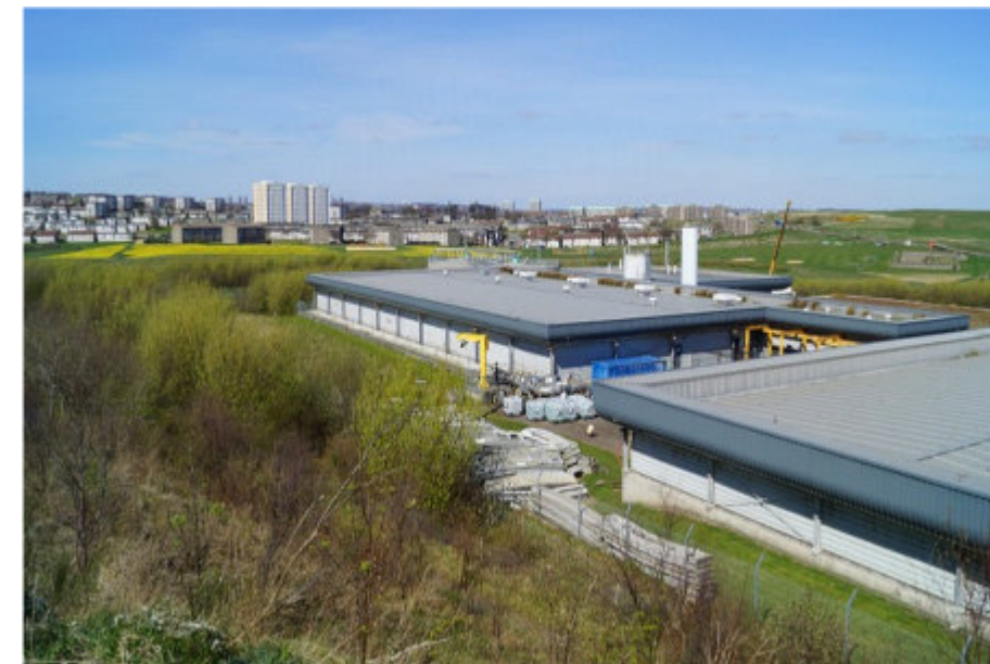
Nigg Waste Water Treatment Works
