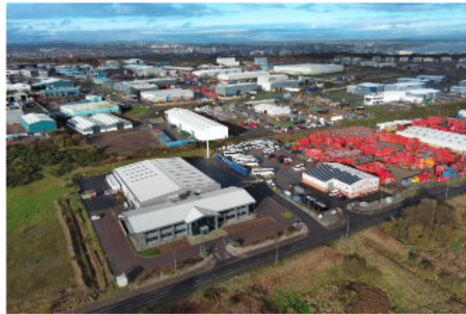
Existing industrial sites and brownfield land should be incorporated with a focus on sustainable retro-fit and re-purposing.
