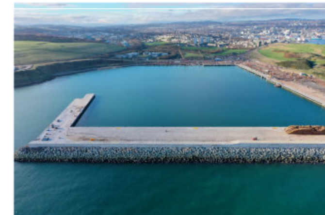
Development should be integrated with Aberdeen South Harbour and provide high-value activity that is a catalyst to further investment across ETZ.
